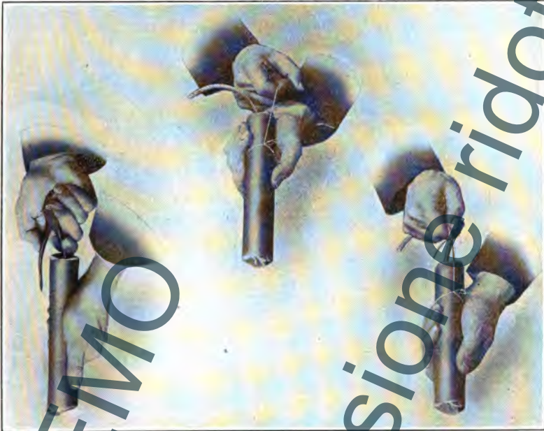
PRIMING IN END OF CARTRIDGE
