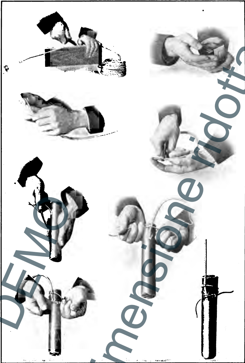
MAKING UP A PRIMER WITH A BLASTING CAP AND SAFETY FUSE
