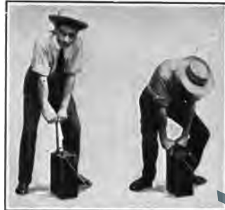
OPERATING A DU PONT BLASTING MACHINE
