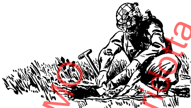
SPOIL BEING REMOVED CORRECTLY
