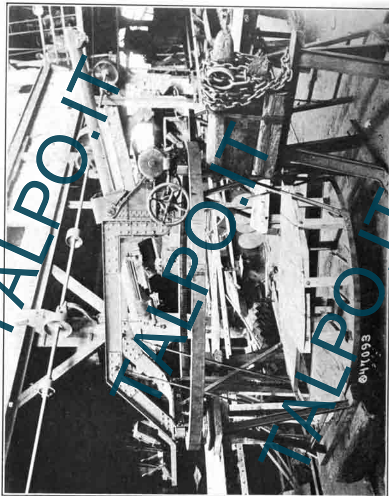
AMERICAN IMPROVED ANTI-AIRCRAFT CARRIAGE, MODEL OF 1917, AFTER IT HAD BEEN CHANGED AND EQUIPPED WITH 75-MM. FRENCH MODEL 1897 FIELD GUN IN FRENCH SHOP. Note changes in platform and change in horizontal supports to riveted U frame to provide better space for loading. (See p. 45.)
