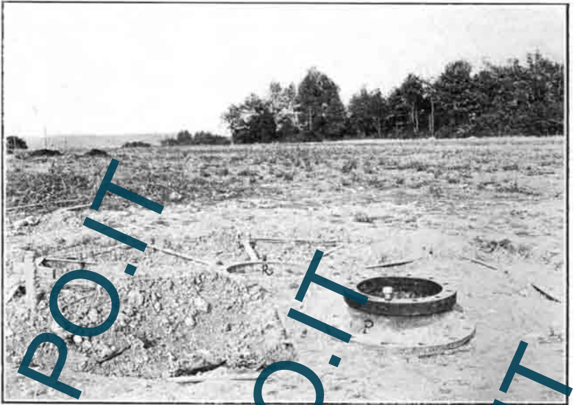
GERMAN SEMIFIXED MOUNT FOR 88-MM. GUN FOR ANTI-AIRCRAFT SERVICE. Note radial bracing from central pedestal mount.
