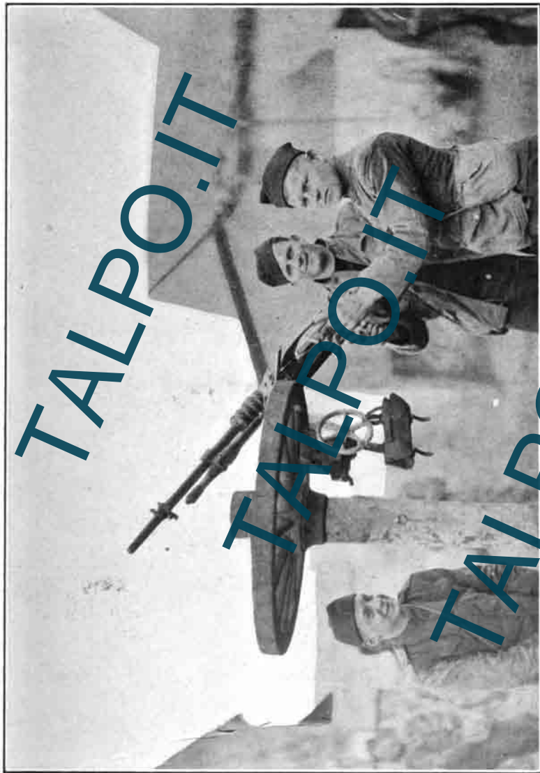
HOTCHKISS MACHINE GUN WITH SERVICE SIGHT, MOUNTED ON RIM OF WAGON WHEEL WITH VERTICAL AXIS. COMBINATION USED AS TEMPORARY EXPEDIENT FOR ANTI-AIRCRAFT WORK, BATTERY E, 6TH FIELD ARTILLERY, MENIL-LA-TOUR, FRANCE, FEBRUARY 17, 1918.
