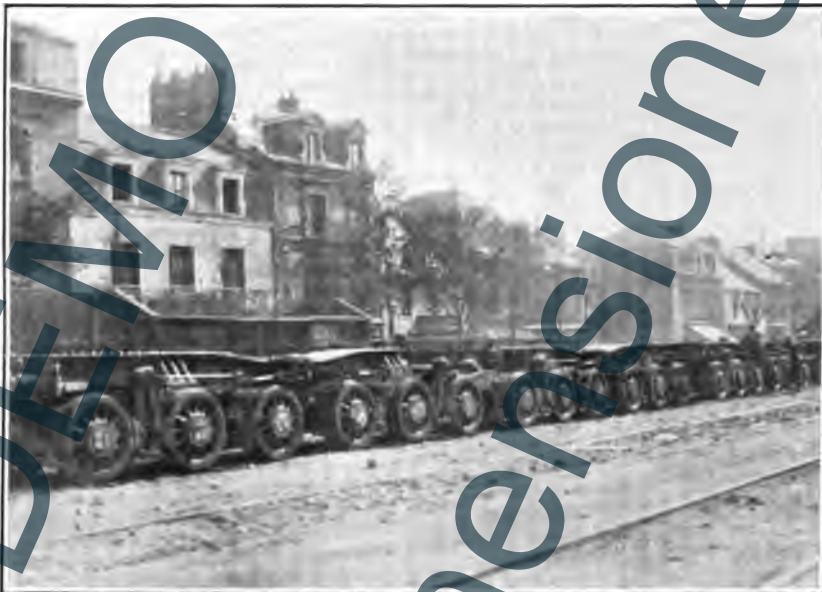
TRUCKS FOR 14-INCH RAILWAY BATTERY GUN CARS LINED UP ALONGSIDE OF DOCK AWAITING UNLOADING OF GIRDEERS.
