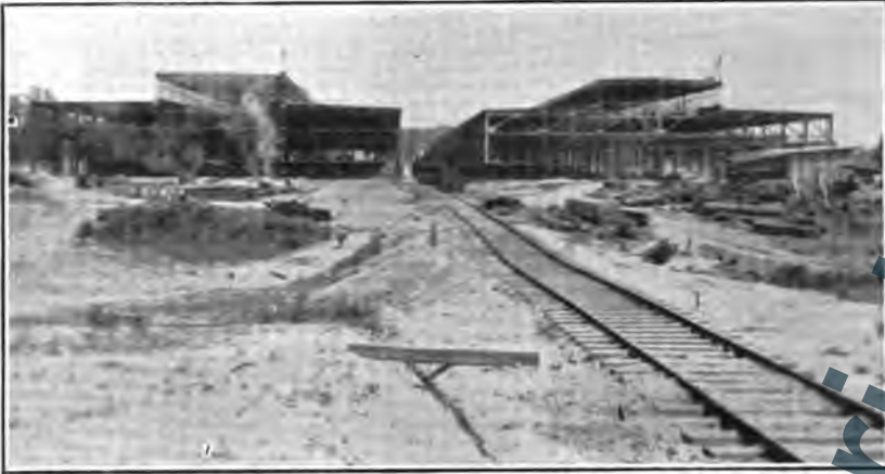
MINE STORAGE BUILDINGS UNDER CONSTRUCTION AT NAVAL MINE DEPOT, YORKTOWN, VA.
