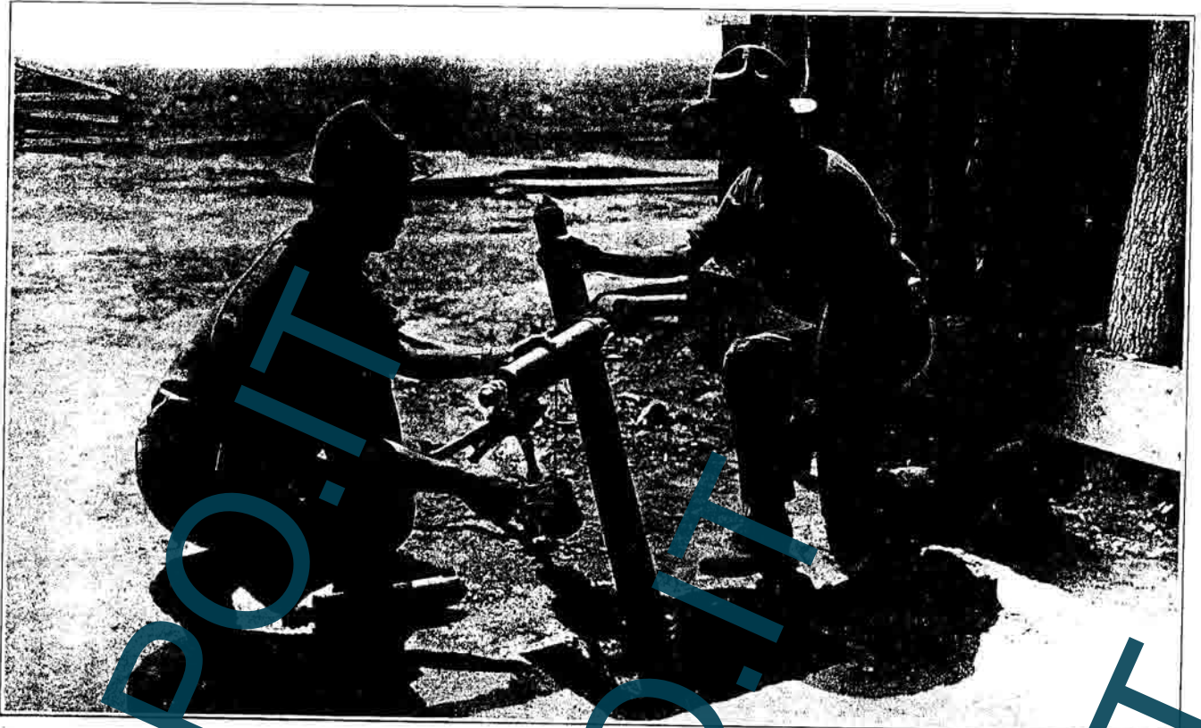
FIG. 95.—3-Inch Stokes trench mortar. Loading for firing. The nature of the projectile can be seen by the shell held by the soldier on the left.
