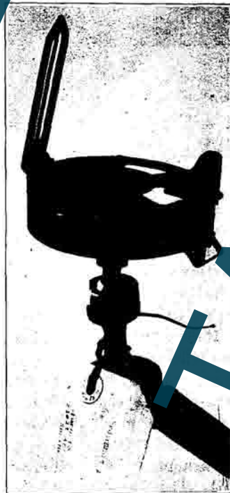
FIG. 145.—Prismatic compass.
